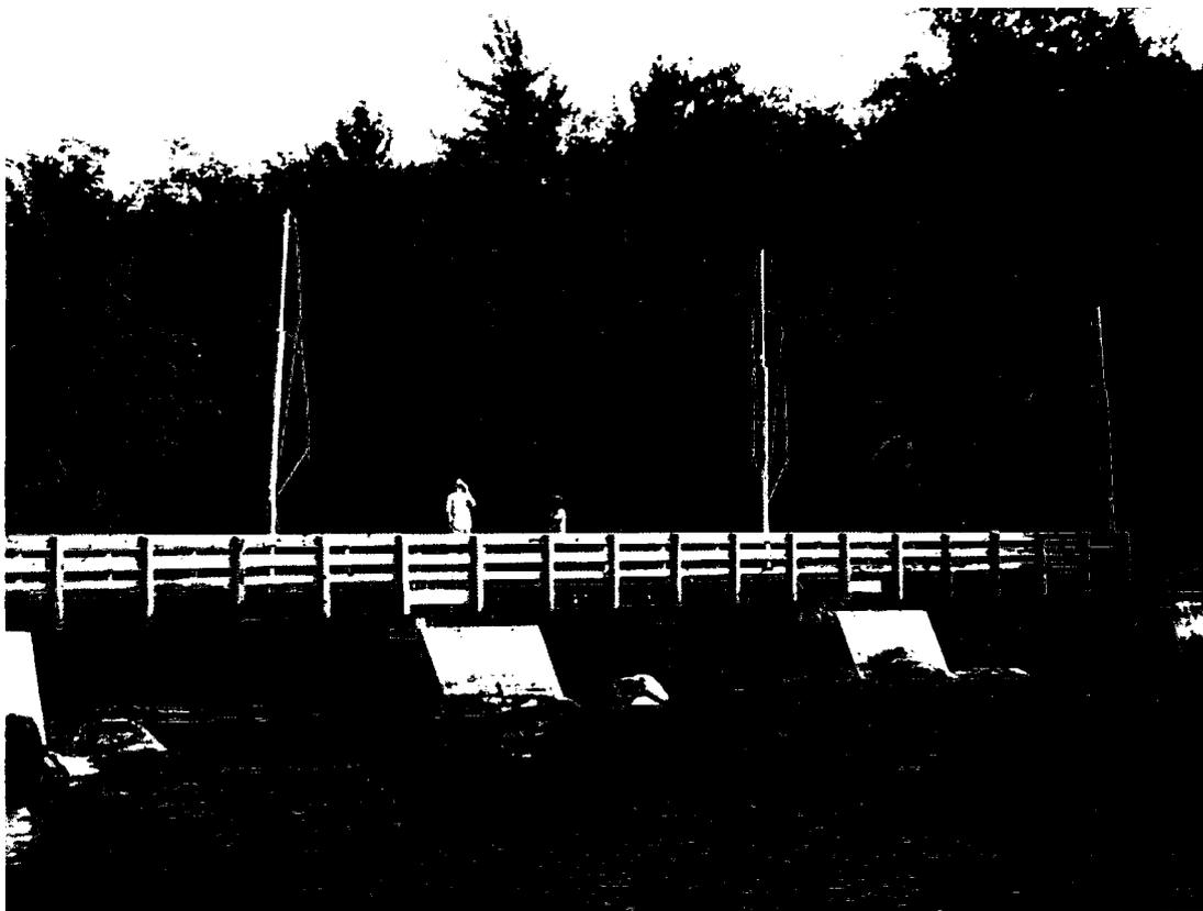
**Figure 4** : Eel Weir site, across the Mersey River in Kejimikujik National Park. Location of intensive trapping effort over four summers, 2003/4 & 2007/8. Tops of masts are 10 m above river. 10 cm x 10 cm lumber with rope and pulley system used to hoist nets.
